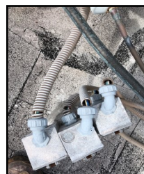
Exposed wiring
